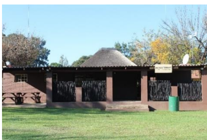
BUDGIE TERRACE – R1,000 Building enclosed with veranda, kitchen/bar, fridge and water points. Equipped with 2 trestle tables, 20 plastic chairs, 20 sitter in-built seats, 1 x drum braai and power point
